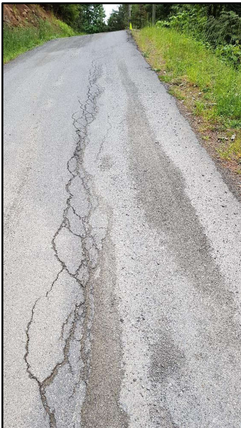
Photo 3 (Left): Paved section of road located uphill from eroded embankment appears to be undermining. Photo 4 (below) looks south at eroded embankment.
