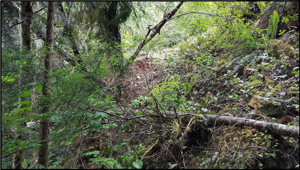
Photo 8: Eroded hillside below gravel road.
