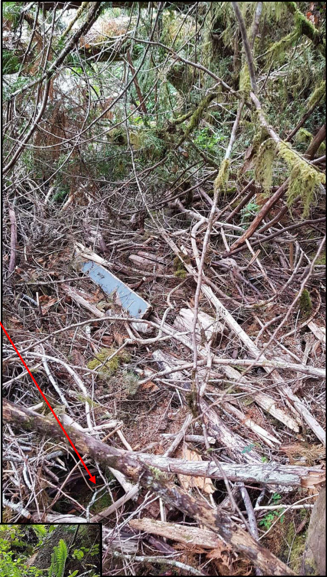
Photo 7: Build-up of wood debris on bank from river flood waters. Area below eroded embankment. Waters edge.
