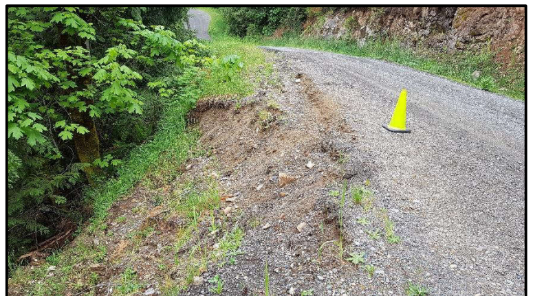
Photo 3 (Left): Paved section of road located uphill from eroded embankment appears to be undermining. Photo 4 (below) looks south at eroded embankment.
